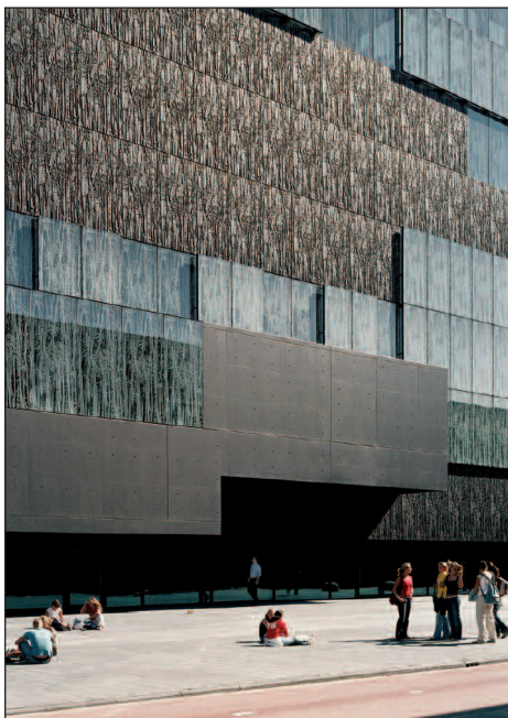
The new university library building, University of Utrecht, The Netherlands
